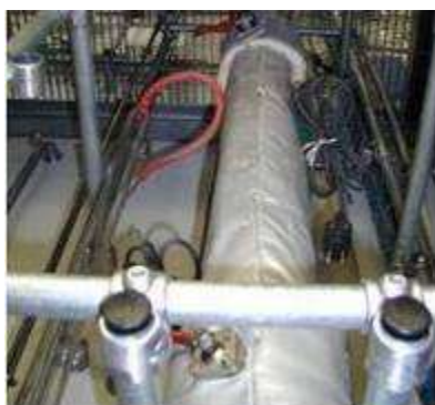
Reactive distillation column – Copyright Rhodia
